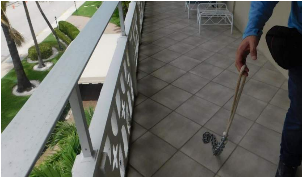
Figure 6. Chain dragging
