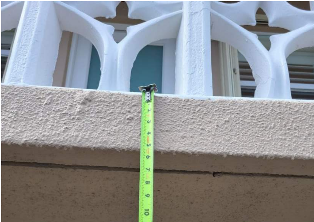
Figure 3. Depth of concrete balcony at slab edge
