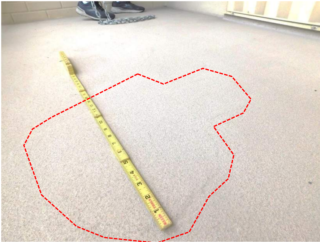
Figure 8. Concrete delamination
