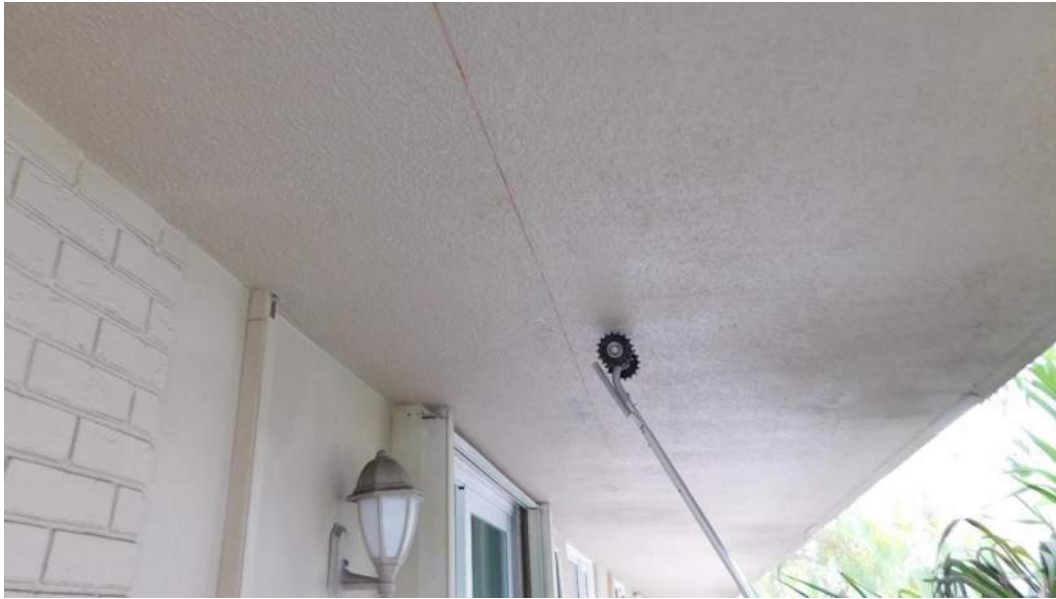
Figure 7. Rotary percussion device to sound the underside of the balconies
