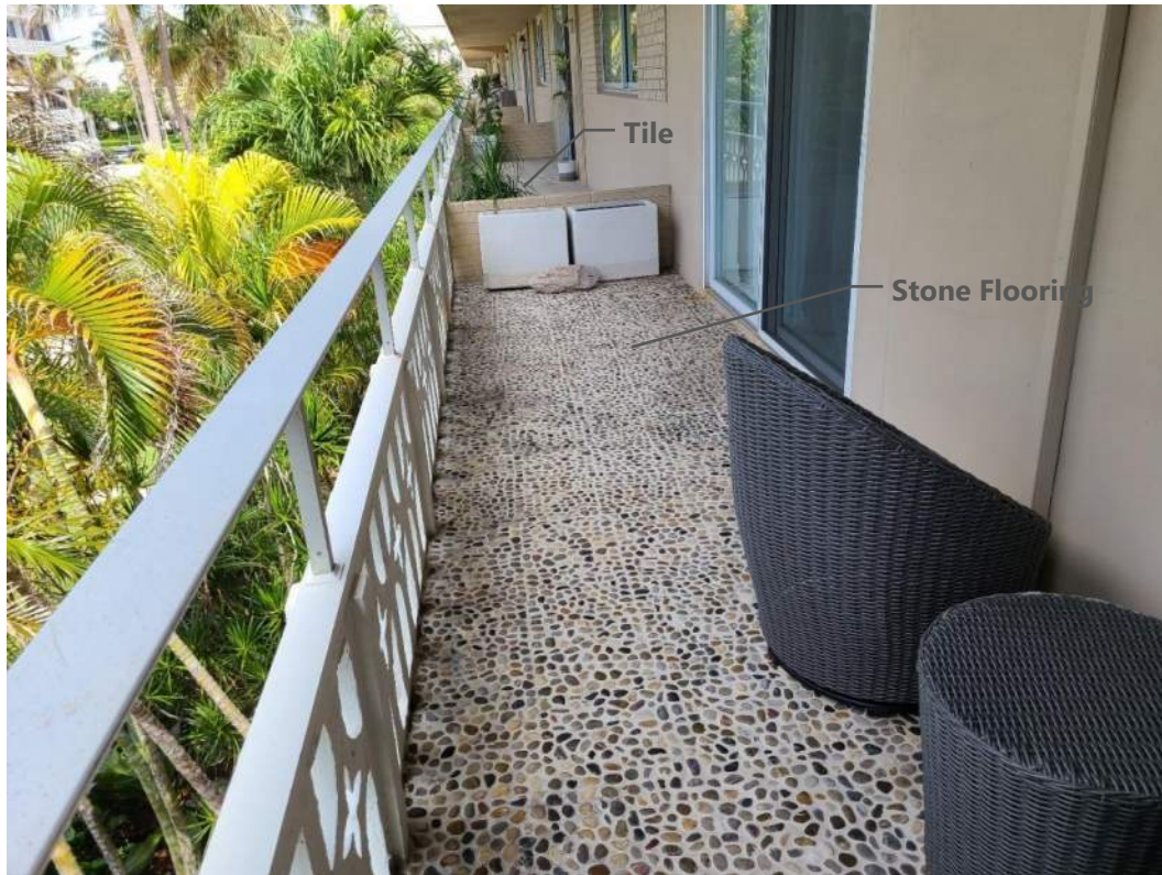
Figure 4. Various balcony finishes observed
