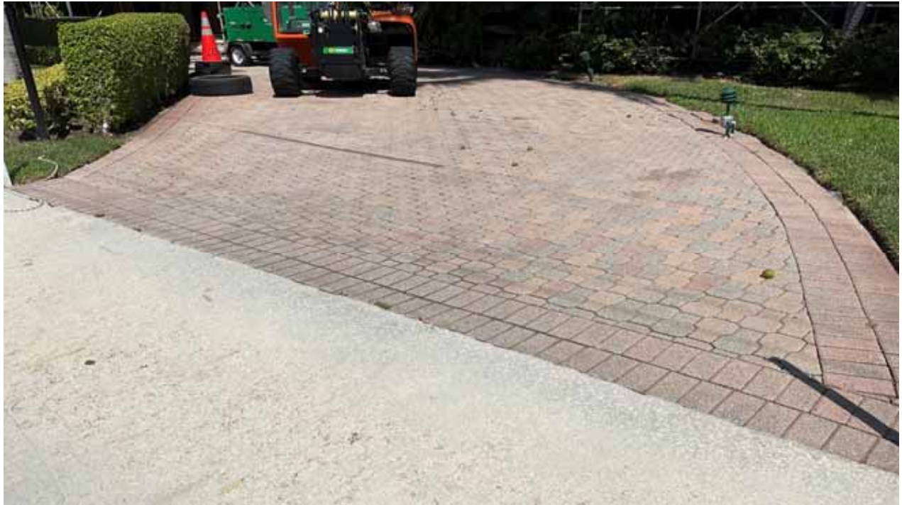
Pavers, South Bldg Entrance - Sunrise Ave
