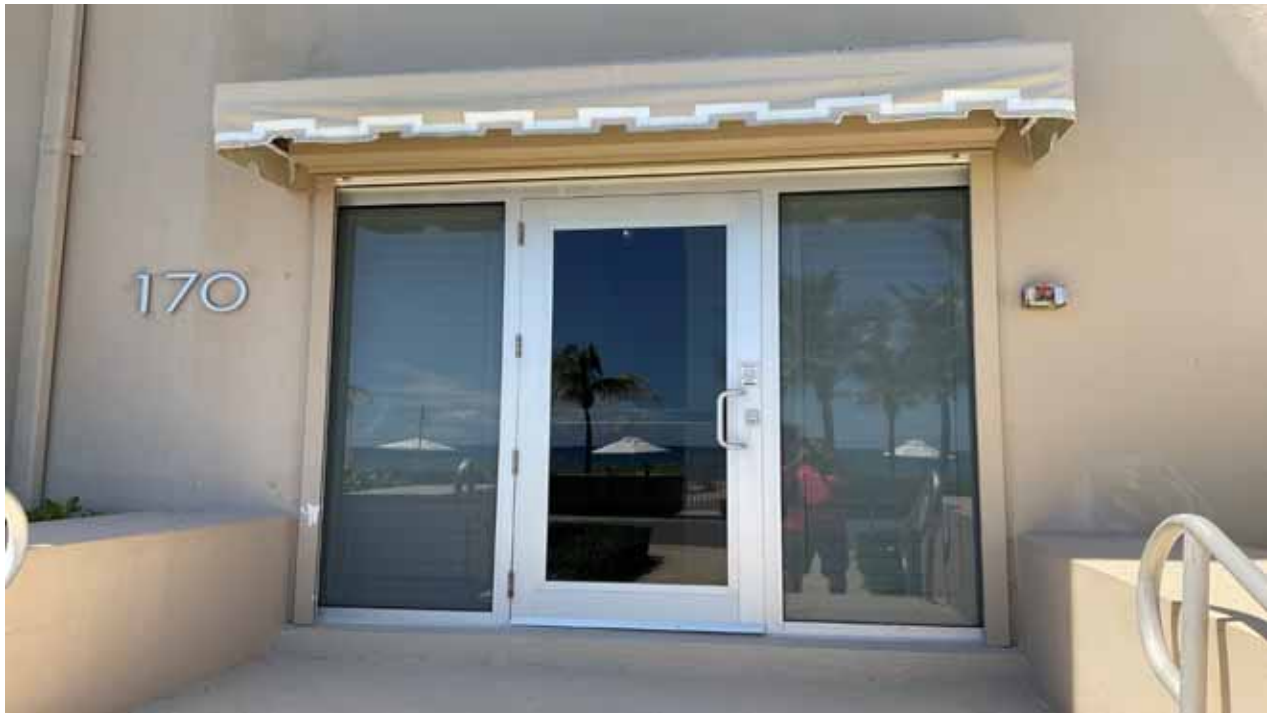
North Bldg East Stairwell Entrance
