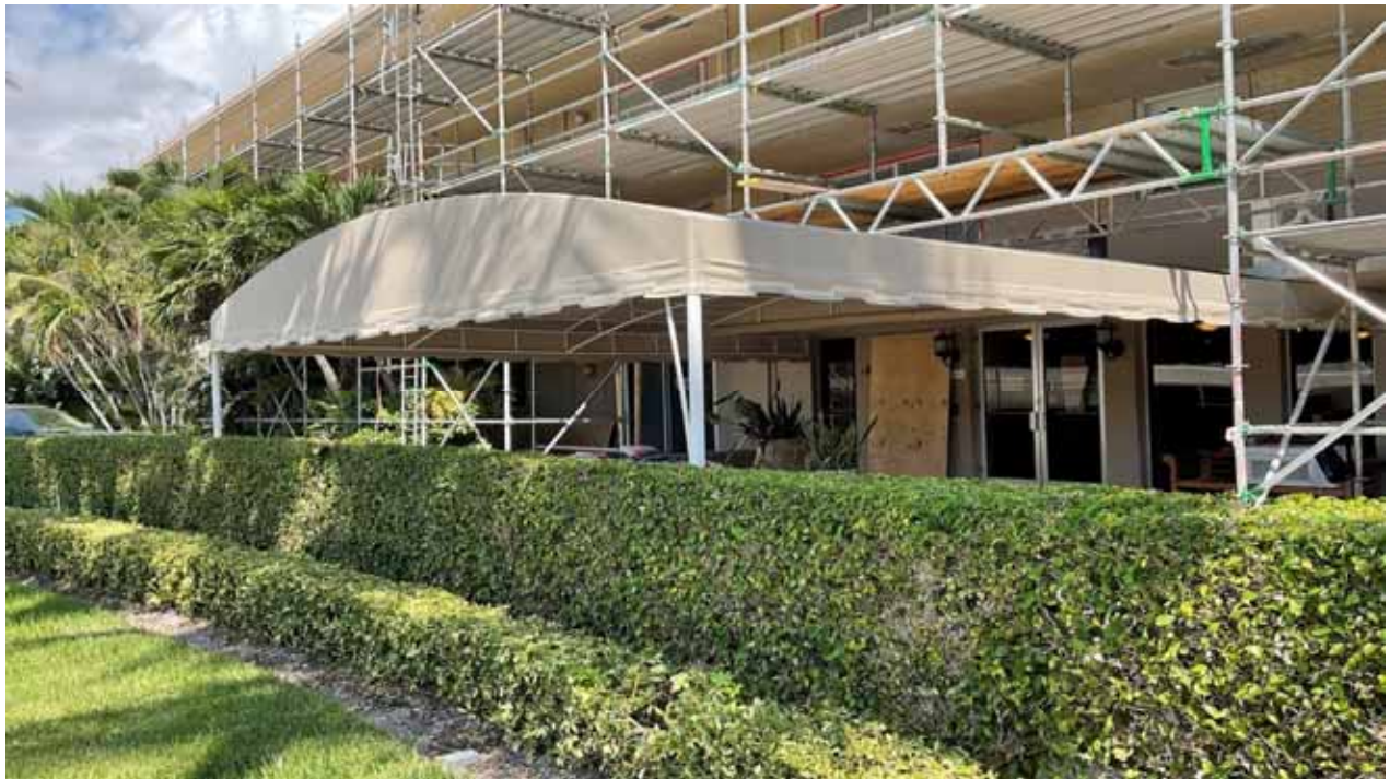
South Bldg Awning, Main Lobby Entrance
