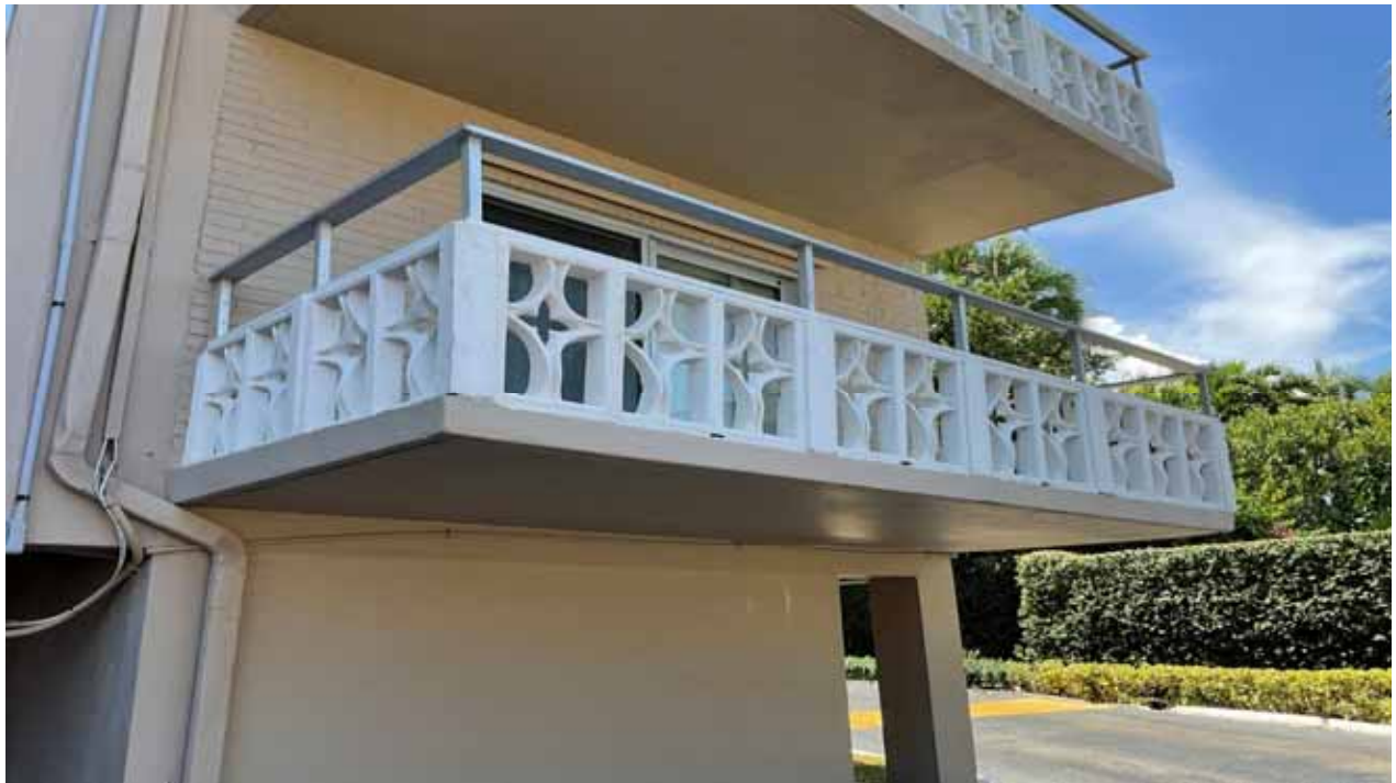
North Bldg Balcony
