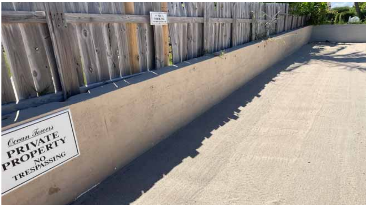
Beach Area Site Wall - South
