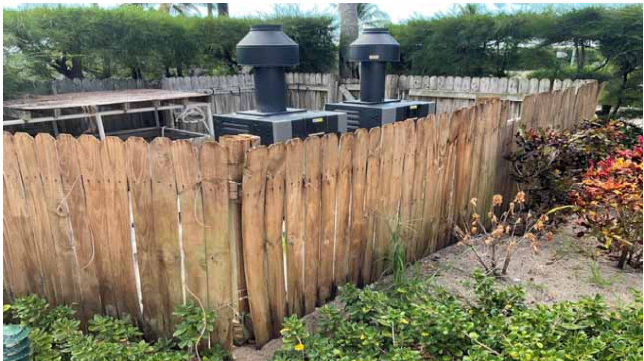
Pool Equipment Fence
