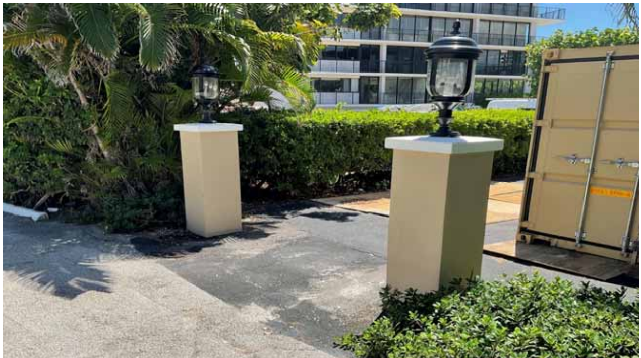
South Bldg Columns & Light Fixtures
