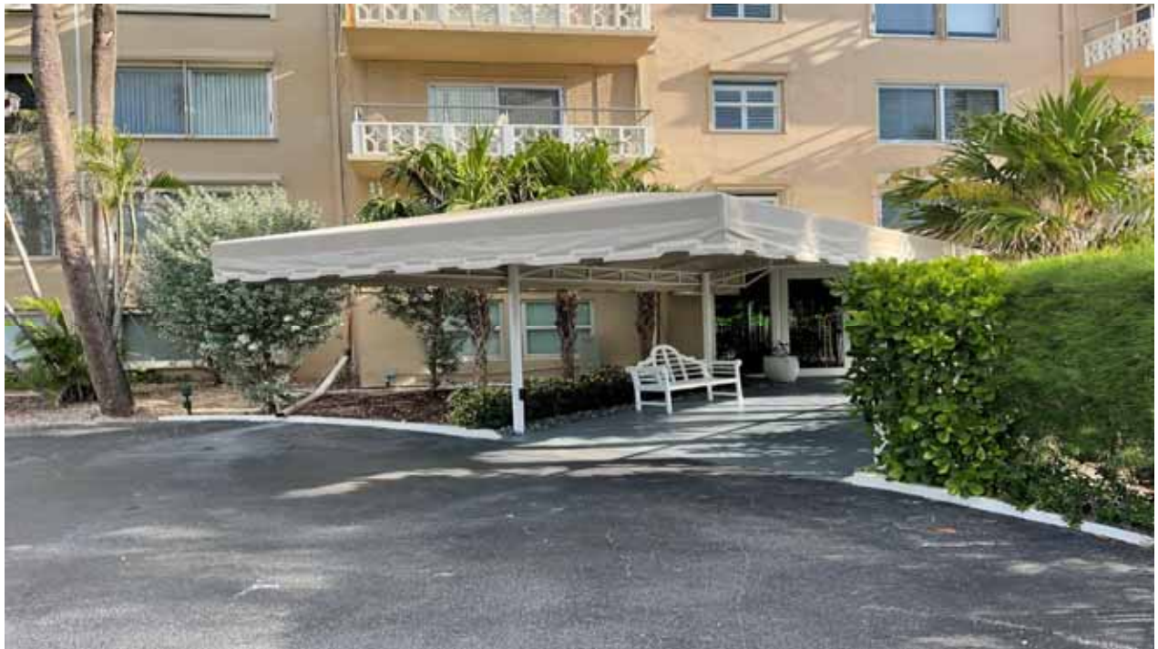
North Bldg Awning, Main Lobby Entrance
