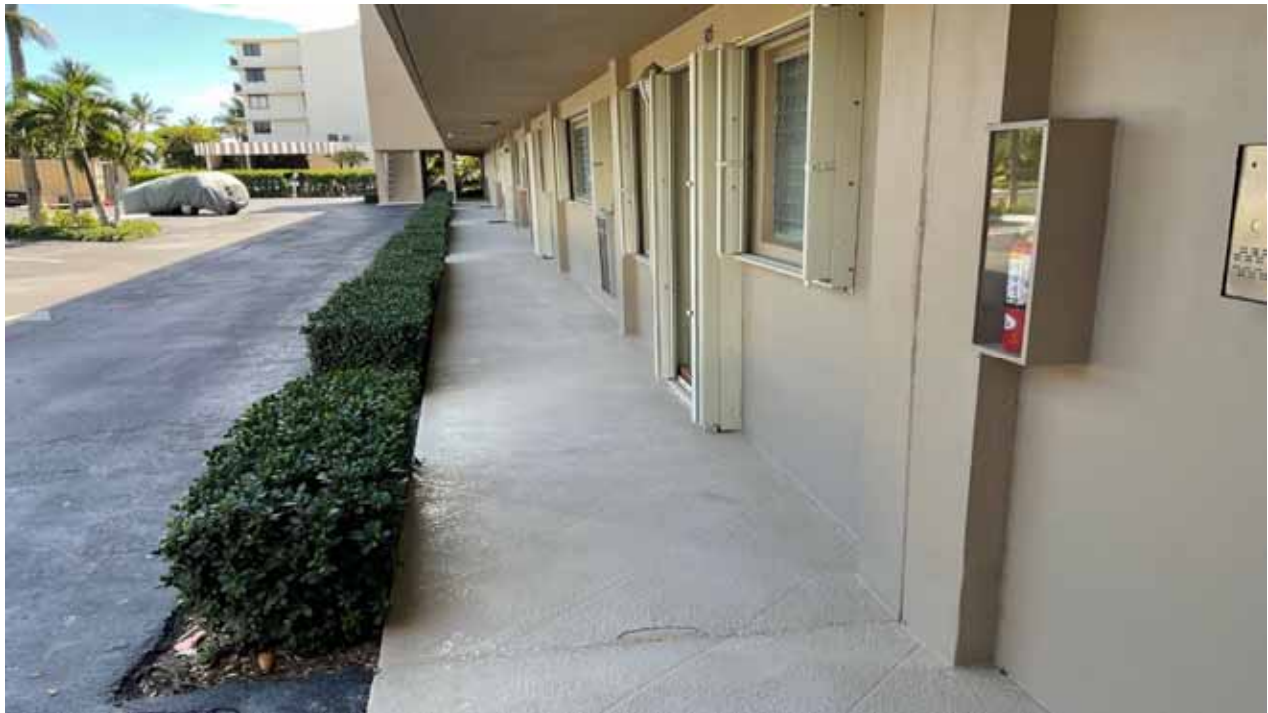
South Bldg Walkway - 1st Floor
