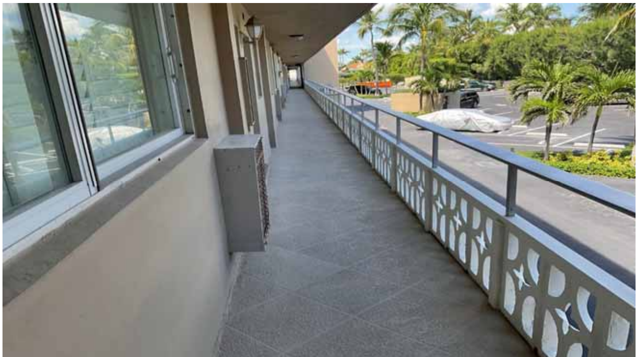
South Bldg Walkway - Upper Floor
