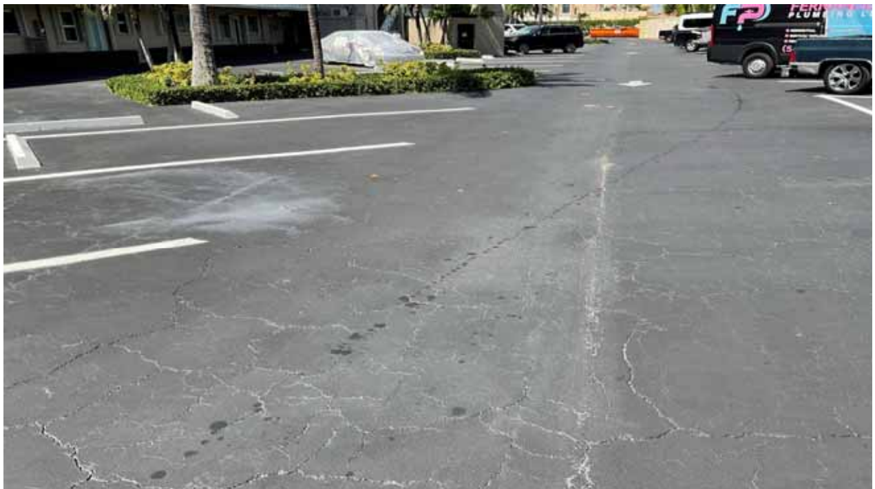
Pavement, Asphalt - South Bldg
