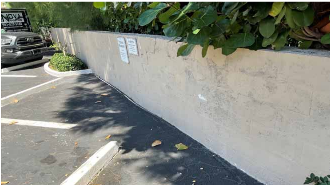
South Bldg Site Wall - North Property Line
