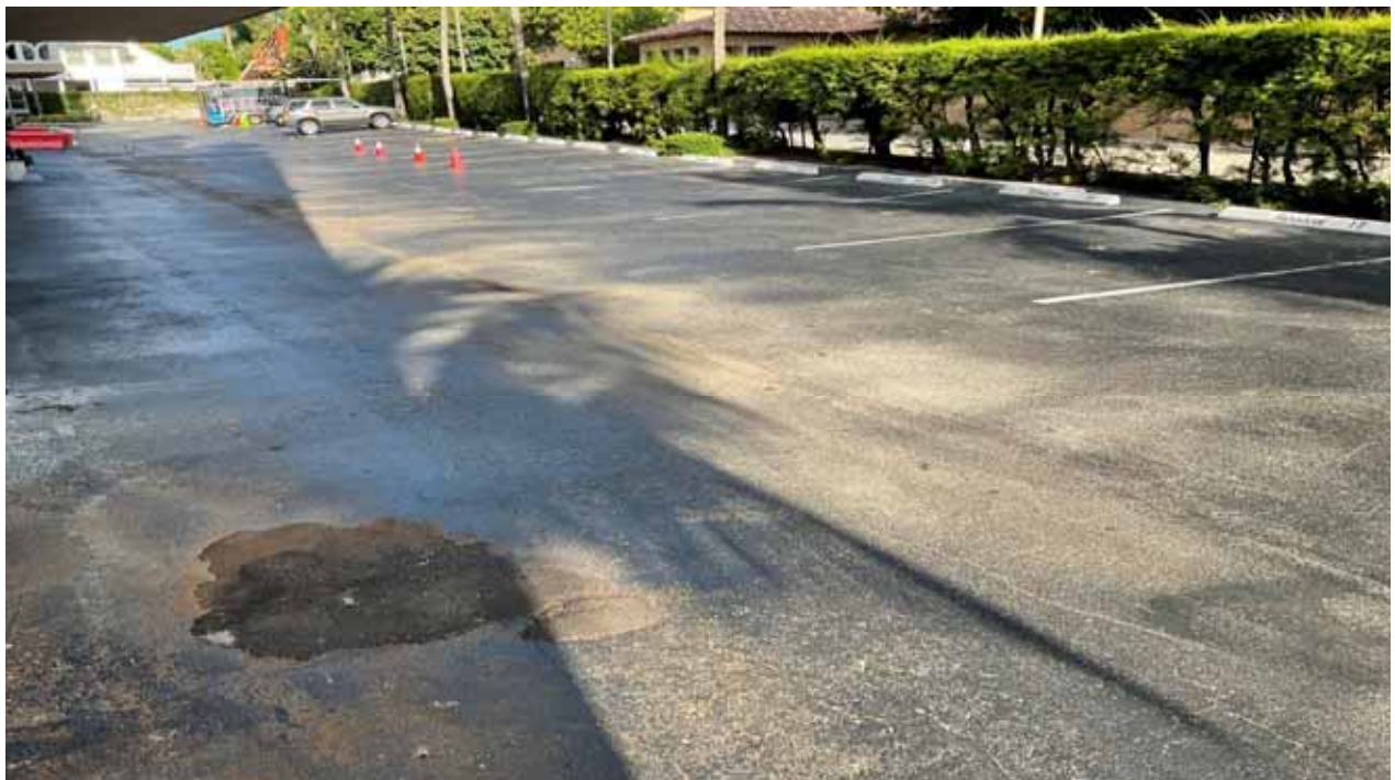
Pavement, Asphalt - North Bldg
