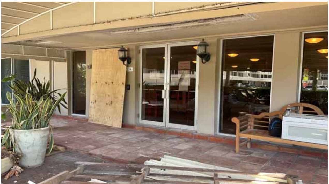
South Bldg Main Lobby Entrance
