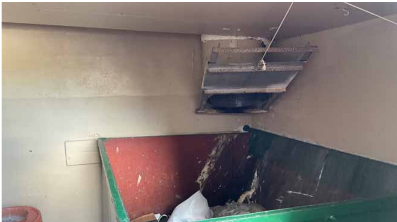
South Bldg Trash Room
