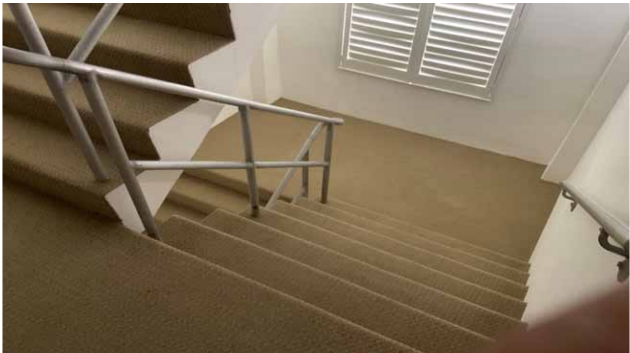
North Bldg Stairwell - East
