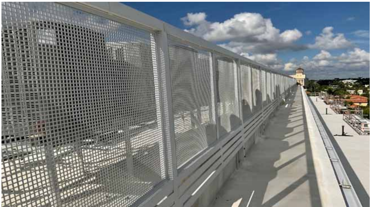
North Bldg Roof Equipment Screen
