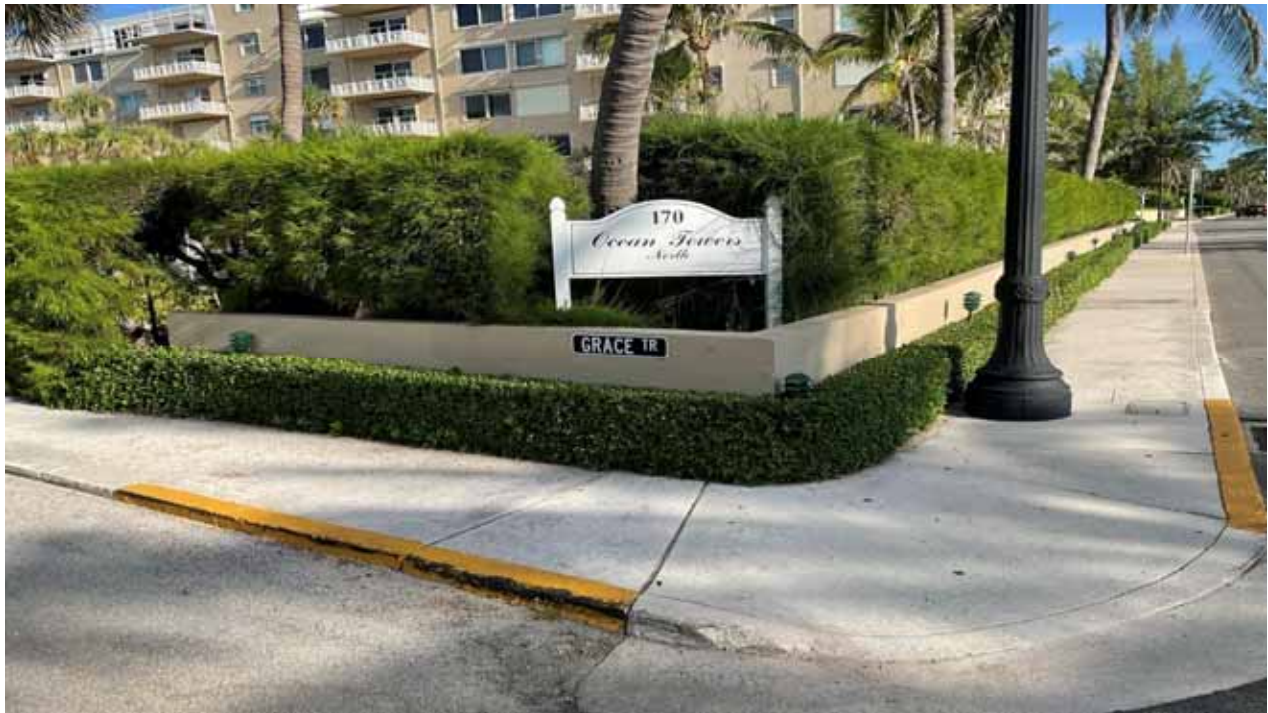
North Bldg Site Wall - East Property Line
