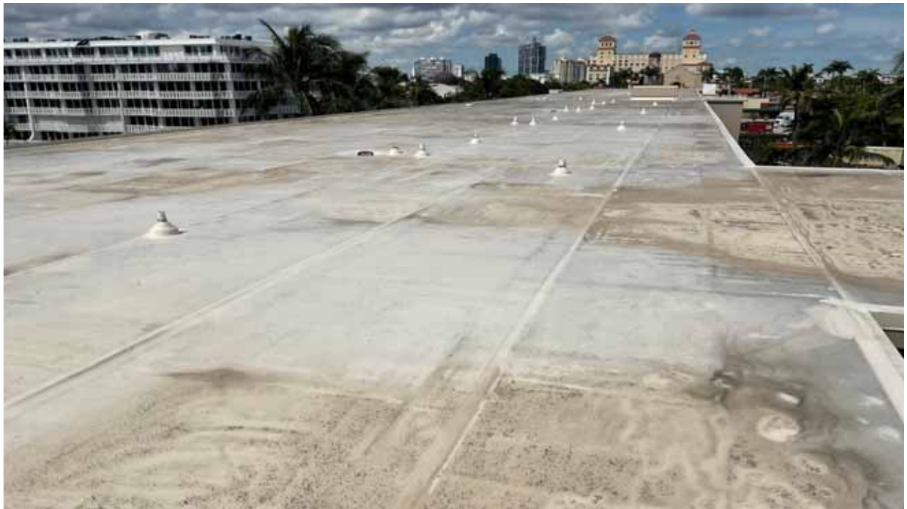
South Bldg Roof
