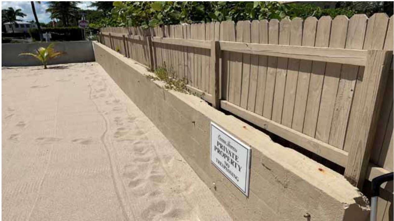
Beach Area Fence & Site Wall - North
