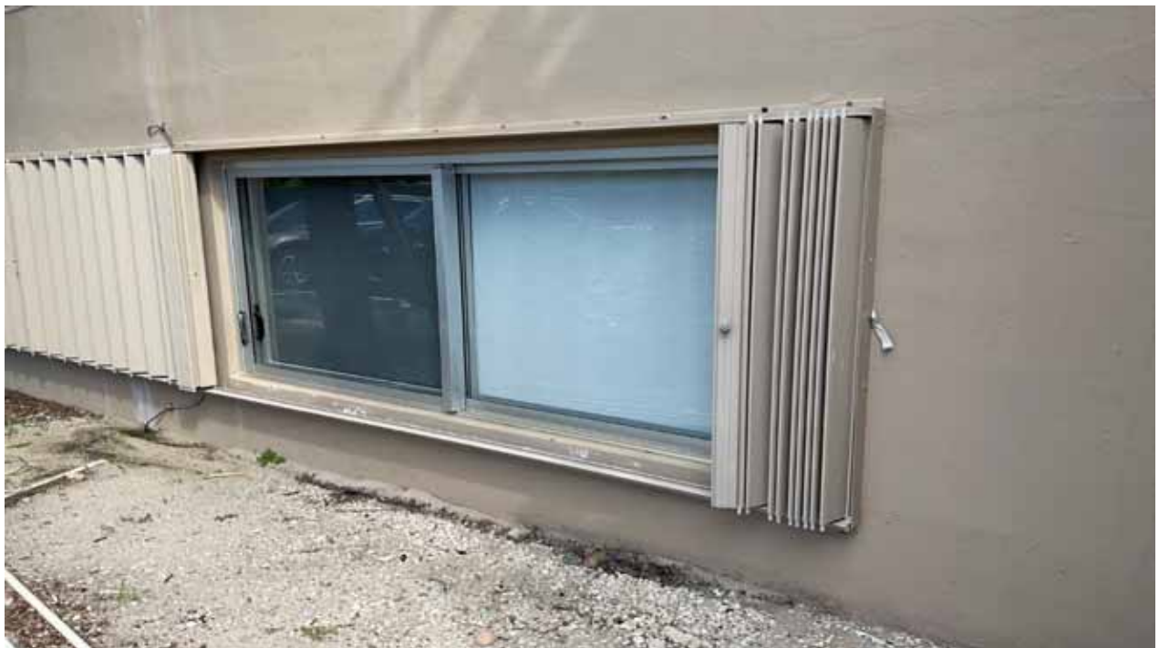
North Bldg Common Area Window & Shutter
