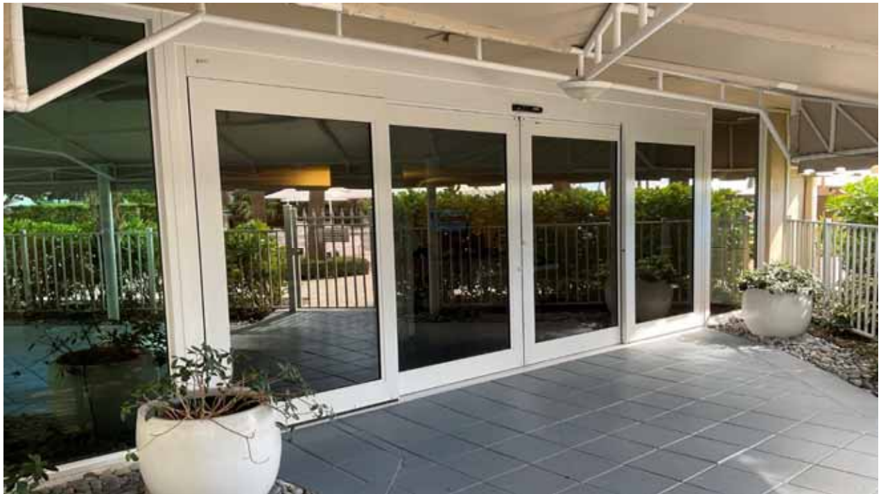
North Bldg Main Lobby Entrance
