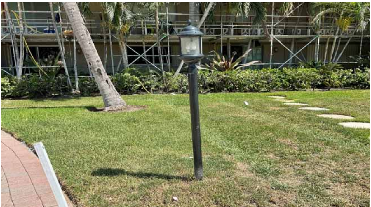
South Bldg Light Pole & Fixture - Sunrise Ave
