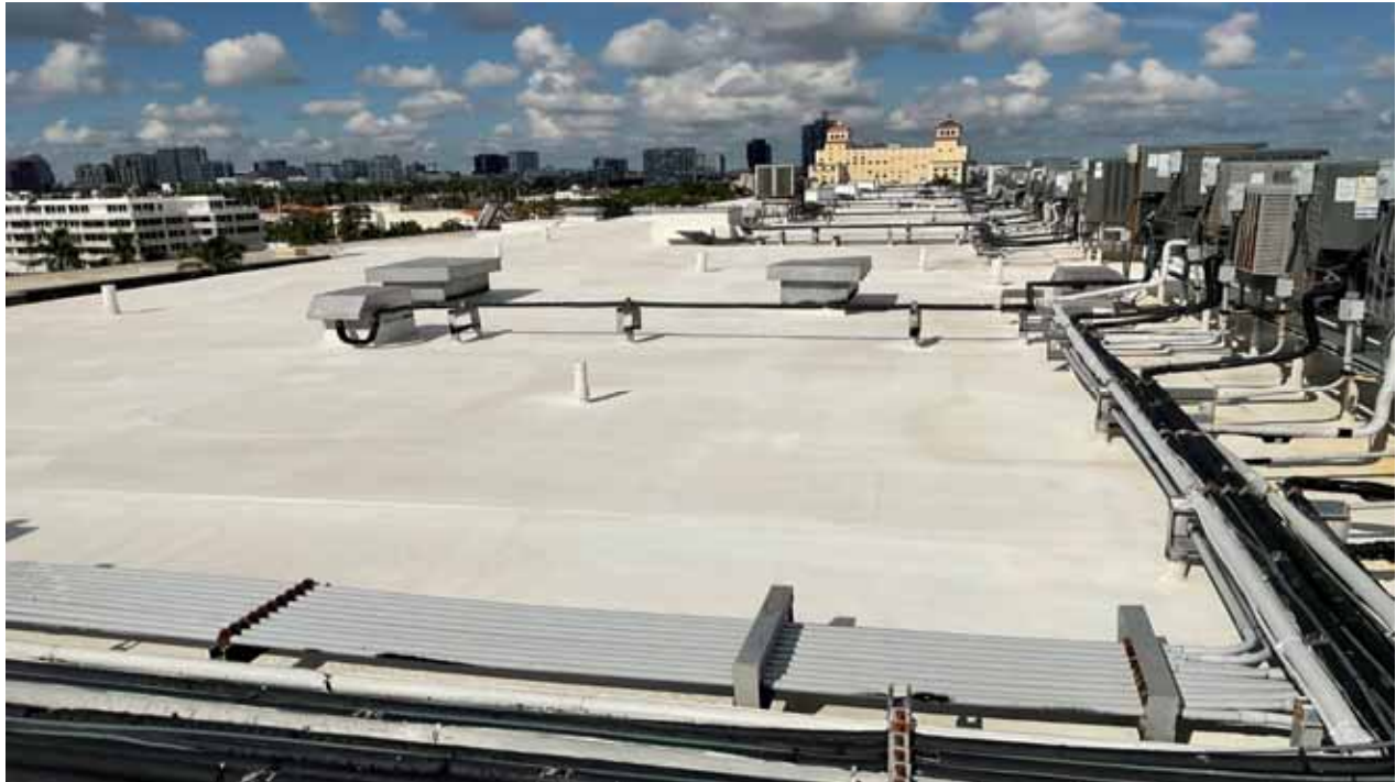
North Bldg Roof
