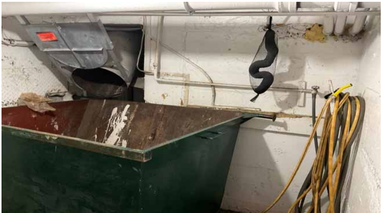
North Bldg Trash Room
