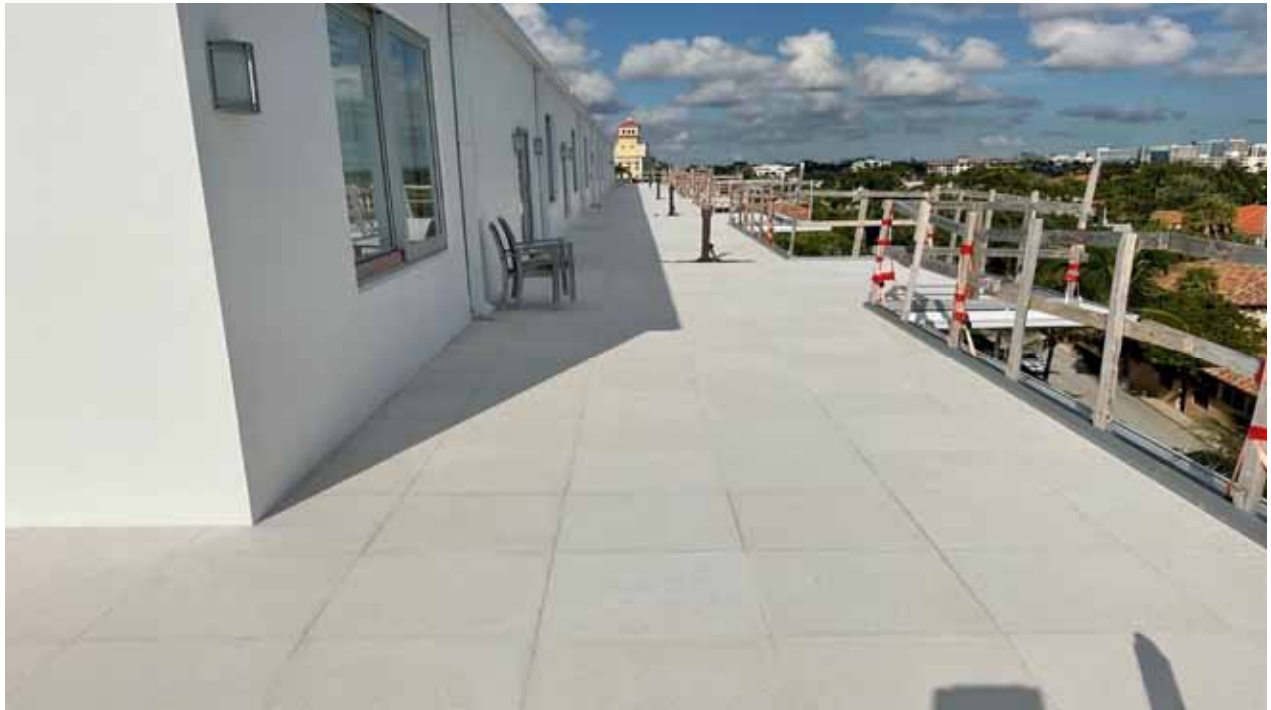
North Bldg Penthouse Terrace Deck
