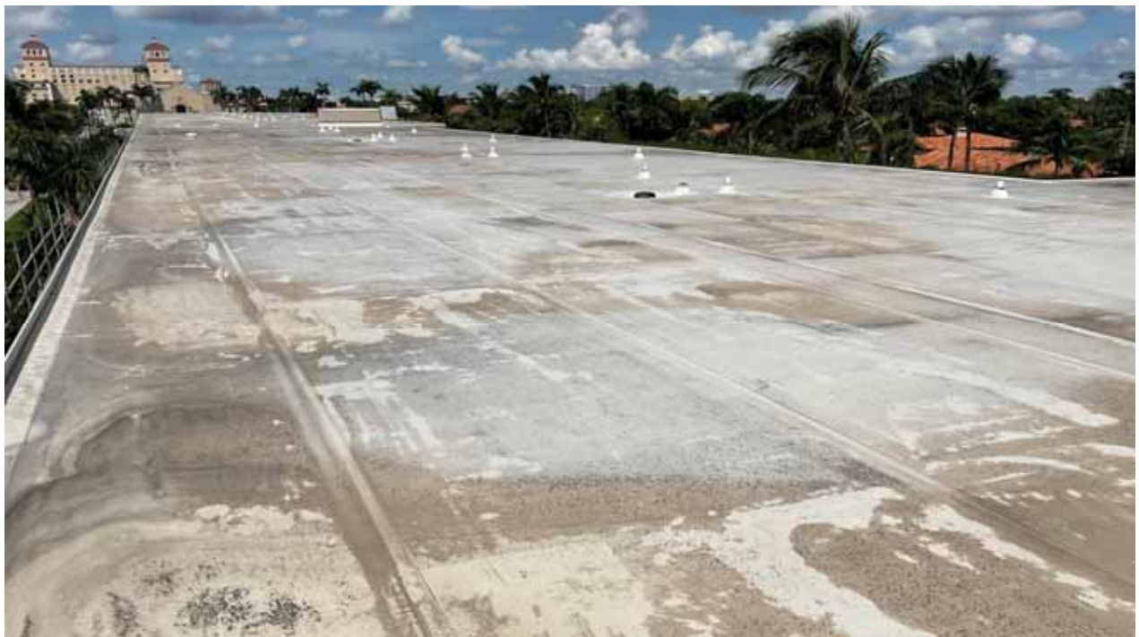
South Bldg Roof
