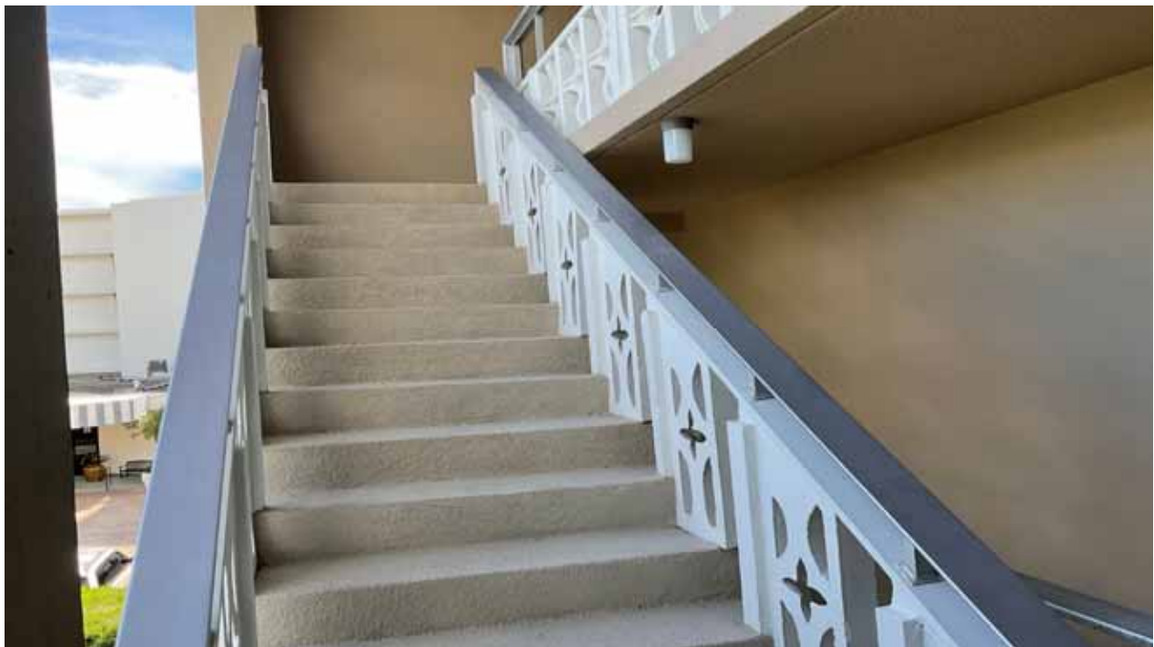
South Bldg Stairway
