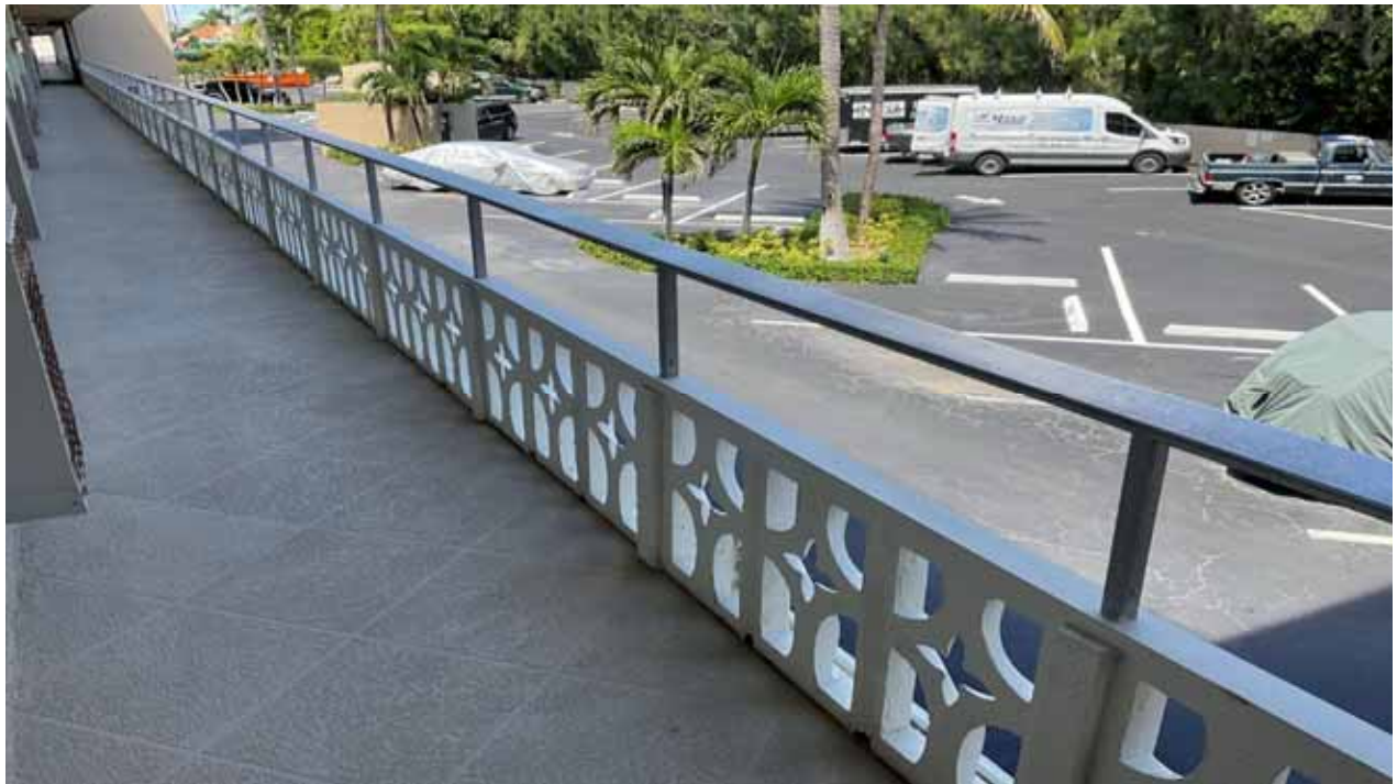
South Bldg Walkway Railing - Upper Floor
